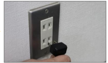
④ If the refrigerator has a power supply, be sure to disconnect the power supply after turning the power off.
