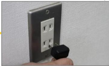
③ Firmly insert the plug of the power cord on the back of the main unit into the dedicated outlet. (Please turn on the equipment with the earth leakage breaker)
