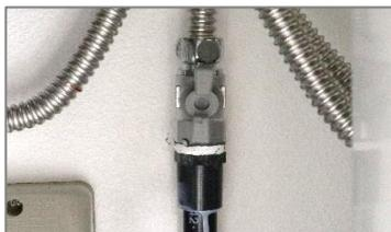
③ Open the water supply valve on the ice maker (Check if there is no water leak)
